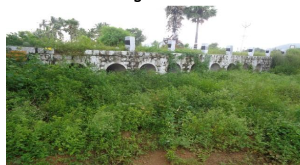
Causeway at km 89/525
