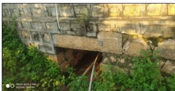
Cut Stone Slab Culvert at Km 6/900
