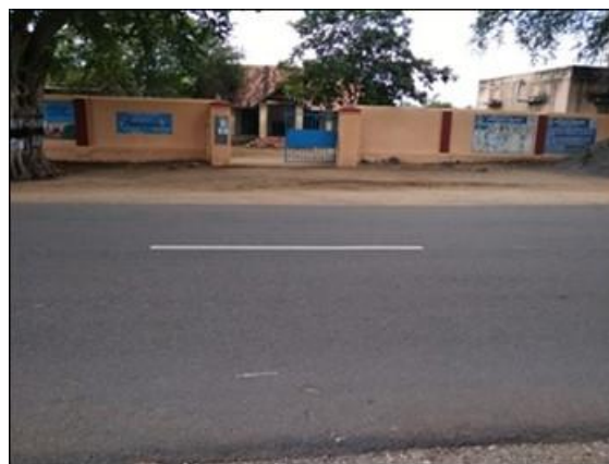
School on RHS at km 82/950
