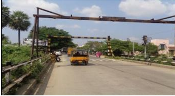
Railway Level crossing at Km 0/250
