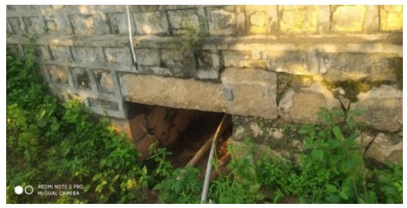
Cut Stone Slab Culvert at Km 6/900
