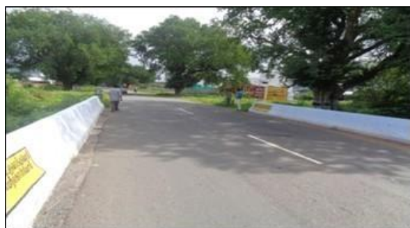
Minor Bridge at km 82/447
