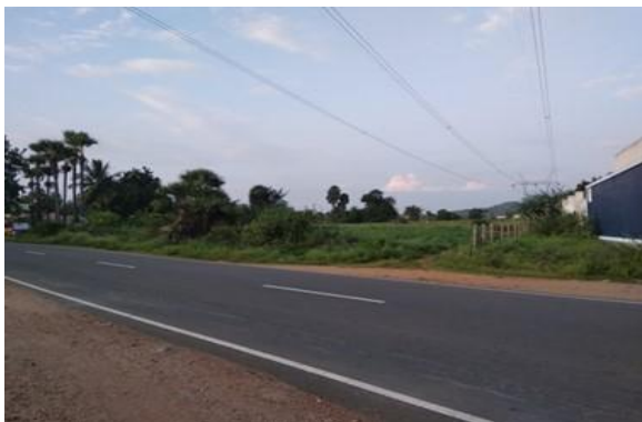
Pylon HT line Crossing at km 9/050
