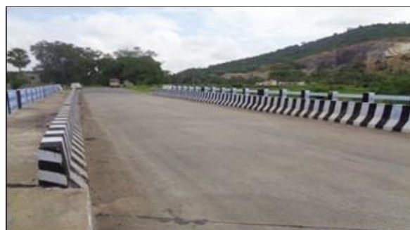
Minor Bridge at km 86/430
