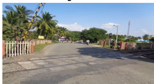
Railway Level crossing at km 90/320
