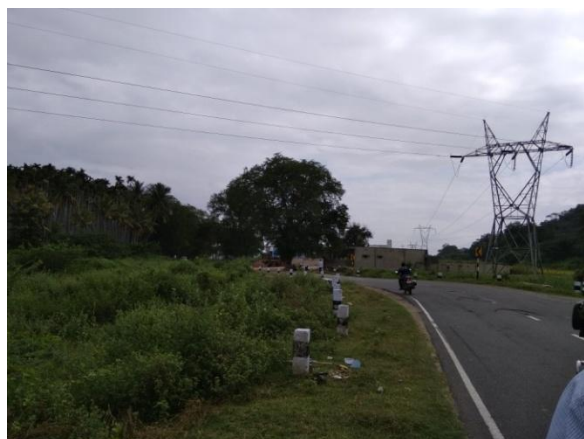
Pylon HT line Crossing at km 86/700
