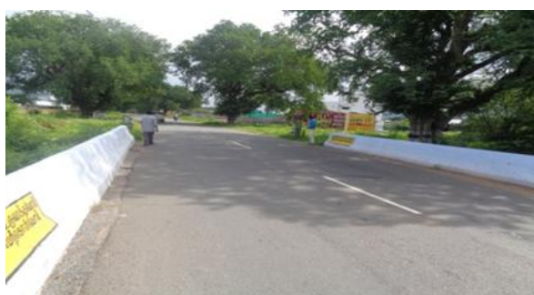
Minor Bridge at km 82/447
