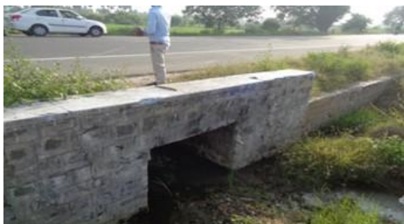
Slab Culvert at Km 154/870
