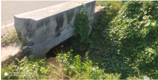
Box Culvert at Km 3/700
