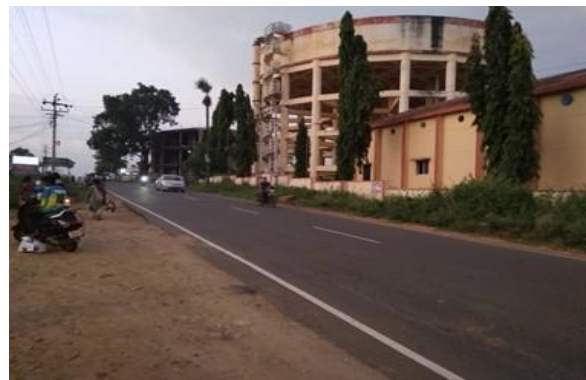
Overhead tank on RHS at km 14/140
