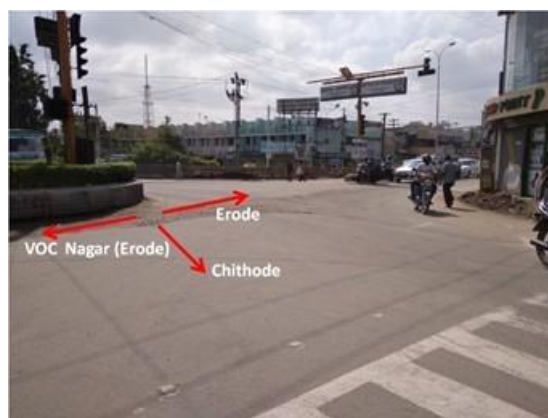
The endpoint of SH 15 (km 161/620)
