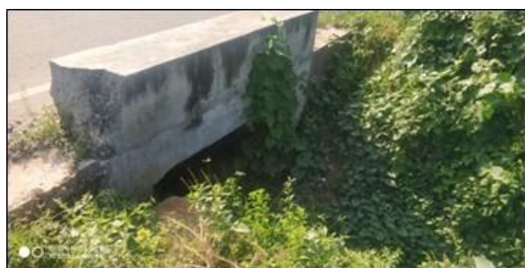
Box Culvert at Km 3/700
