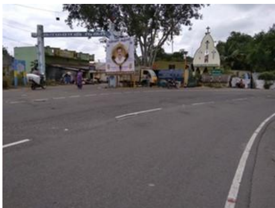
Church on RHS at km 88/060
