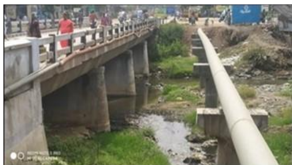
Minor Bridge at km 159/215
