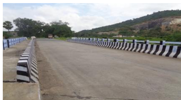
Minor Bridge at km 86/430
