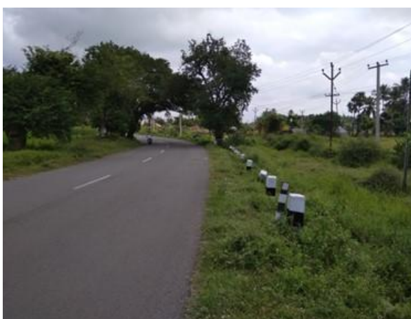
Avenue Plantation between km 89/000 to km 90/000
