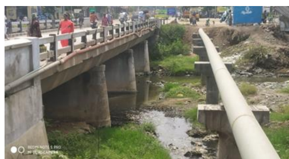
Minor Bridge at Km 159/215
