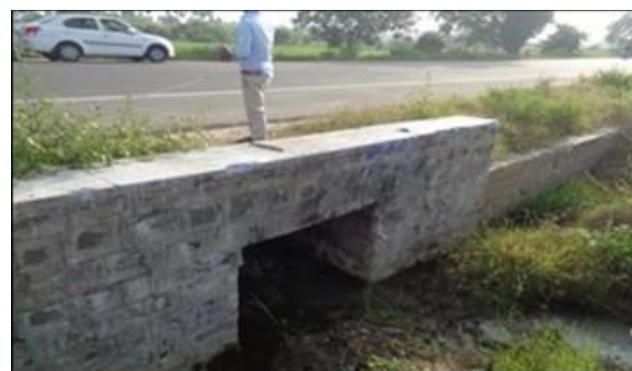
Slab Culvert at km 154/870
