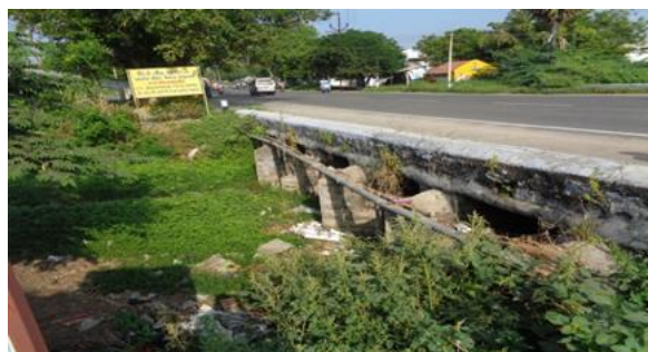
Minor Bridge at Km 156/230
