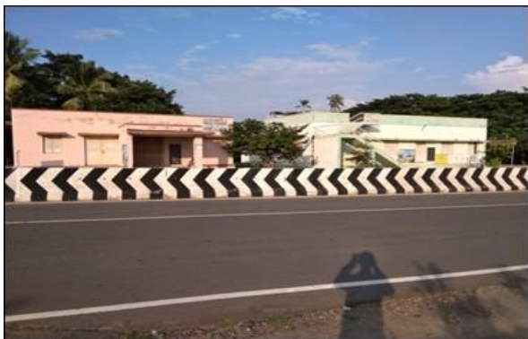
Hospital on LHS at km 3/810
