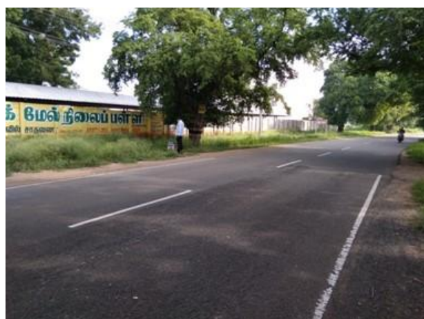
Avenue Plantation between km 82/000 to km 83/000
